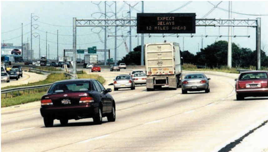
FIGURE 3-14 A dynamic message sign. SOURCE: Delaware Department of Transportation.
