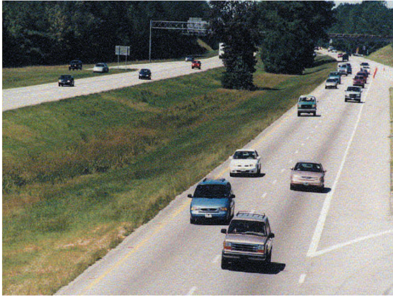
FIGURE 3-22 Contraflow along I-26 near Charleston, South Carolina, during reentry after Hurricane Floyd in September 1999. SOURCE: South Carolina Department of Transportation.
